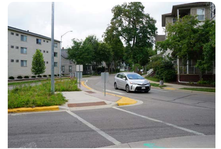
At Bassett and Wilson, crossing improvements such as continental markings, "Yield to Pedestrians" signs, and lighting improve pedestrian comfort and safety.
