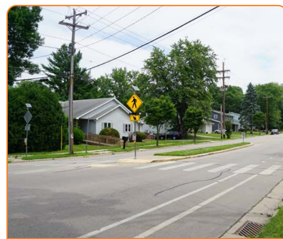
RRFB installed at Milwaukee St. at Swanton Rd., located in a RESJI/Equity Focus Area
