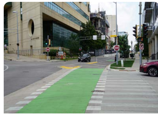
At Wilson, Henry, and Hamilton, raised crossings, pavement markings, and bike signals put cycle track and sidewalk users first.
