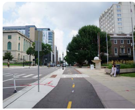
Watch for bikes and cars! Tactile blocks are used at crosswalks, while directional blocks are used beside the cycle track.
