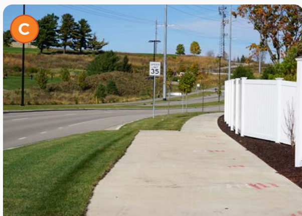
Figure C: Bike ramps allow cyclists to enter and exit the road when approaching an intersection crossing, similar to a freeway ramp.
