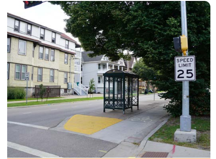
Floating bus stops allow buses to stay in their lane and improve boarding for disabled passengers. These can be found along S Bassett and S Broom Streets.
