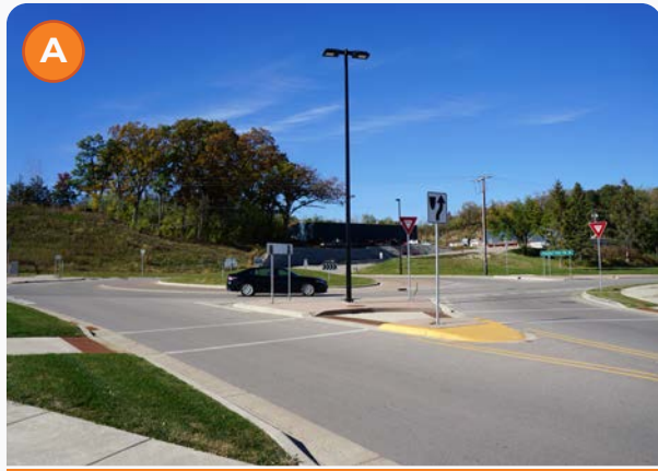
Figure A: Refuge Islands at roundabouts and lighting improvements keep path and sidewalk users visible and comfortable.
