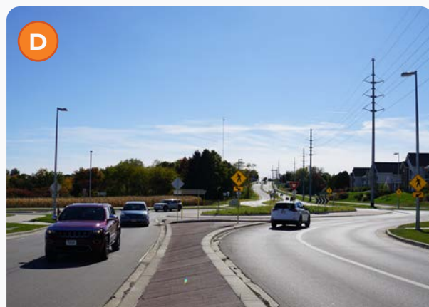
Figure D: Roundabouts, curved roads, and medians all help calm traffic and encourage drivers to maintain the speed limit.
