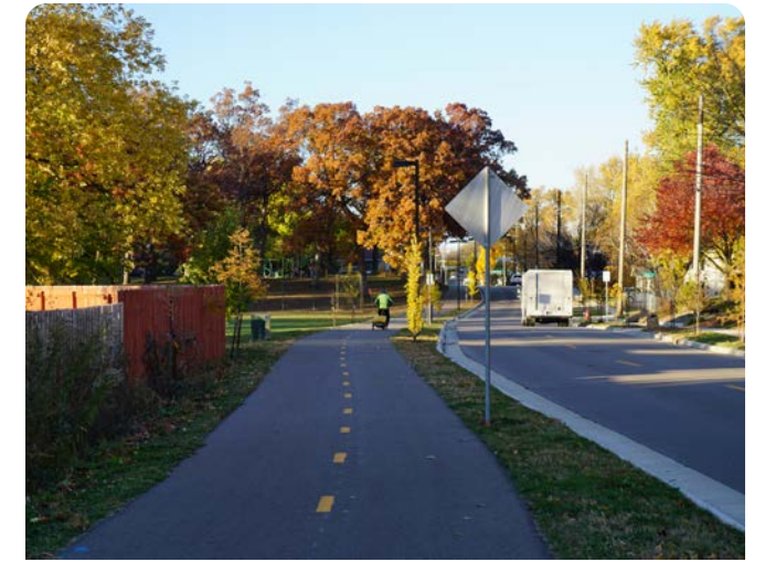
Prior to 2023, Dempsey Rd. and Davies St. lacked sidewalks or dedicated bikeways. Now, the corridor connects the neighborhood to the rest of Madison's active transportation network.
