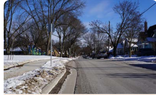
The narrowed street makes way for a new sidewalk and slows car traffic down.
