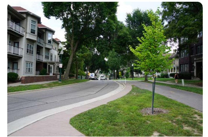
Road diets on Wilson and Broom made room for two bi-directional cycle tracks, accompanied by sidewalks.
