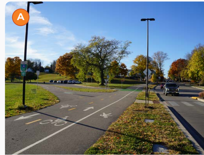
Figure A: Lake Loop connection via separated shared-use path and improved crossing.
