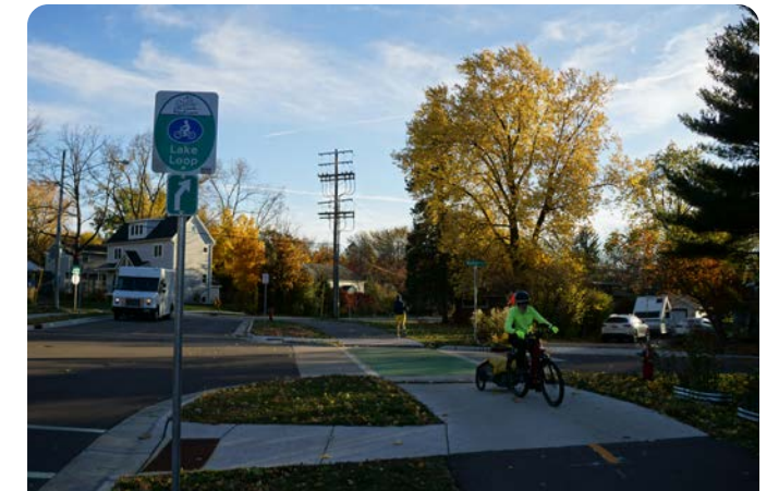
Raised crossings along the new shared-use path improve bike and pedestrian safety and comfort while making path users more visible to cars.
