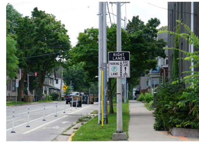
Parking-protected bike lanes were installed along Bassett St. to add an extra layer of protection for bikes headed east.
