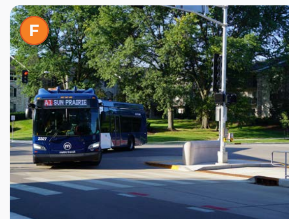
Figure F: Leading Pedestrian Intervals (LPIs) and median islands create a safe environment for riders and pedestrians.
