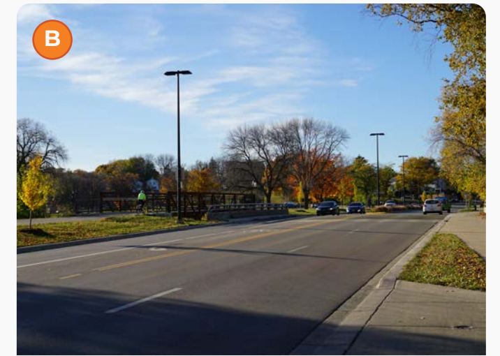
Figure B: Separated shared-use path bridge and lane reductions on Atwood Ave.
