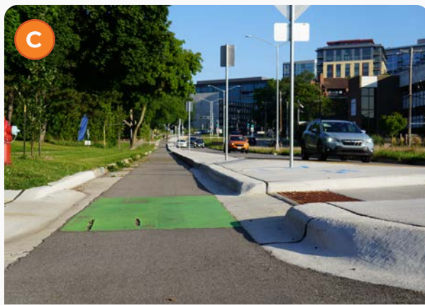
Figure C: Protected bike lanes and curb extensions improve visibility for pedestrians at Heather Crest and Segoe Road.
